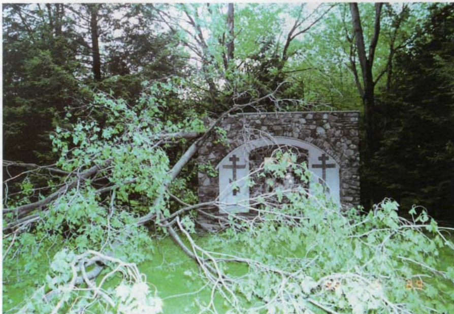
Damage sustained by the shrines.
