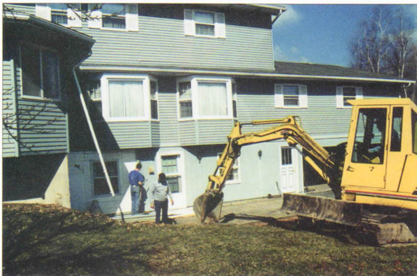
Construction at Diocesan Center
