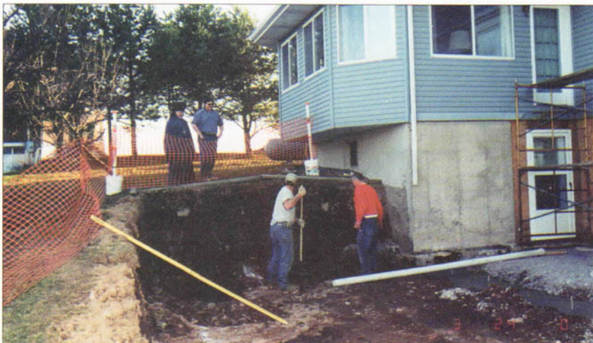
Archbishop Herman inspects progress on the construction
