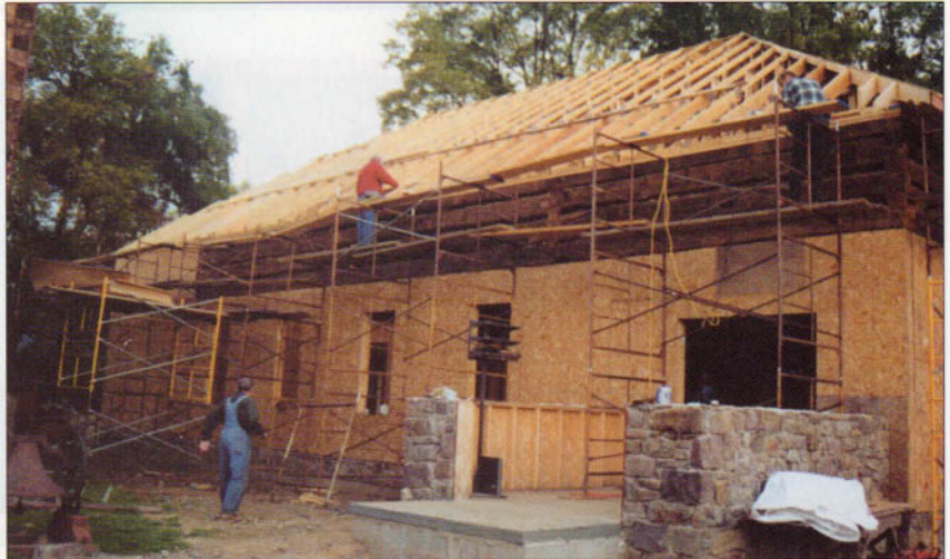
Building the roof of new fellowship center at Holy Cross
