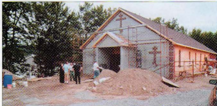
Archbishop Herman inspects construction of new church
