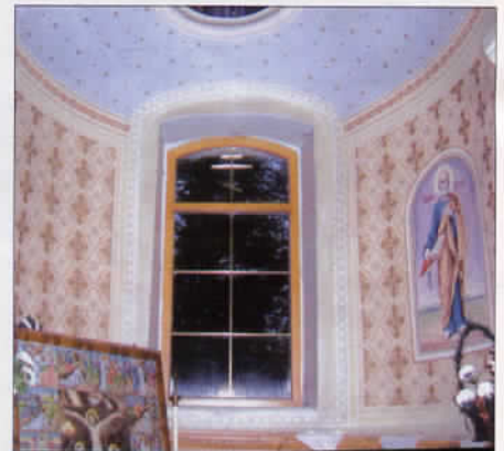
New windows installed
